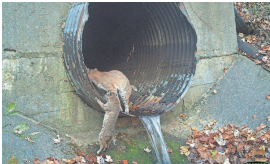
With few exceptions, most drainage structures used in highway construction near the Smokies are too small, too dark, or too wet to be used by bobcats.
